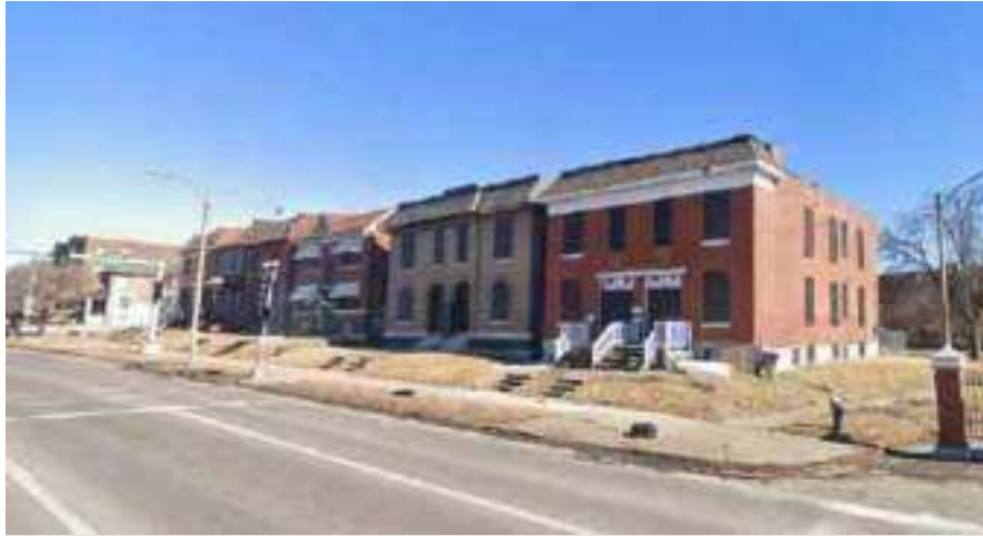
S Kingshighway View of Site (Before Demolition)
