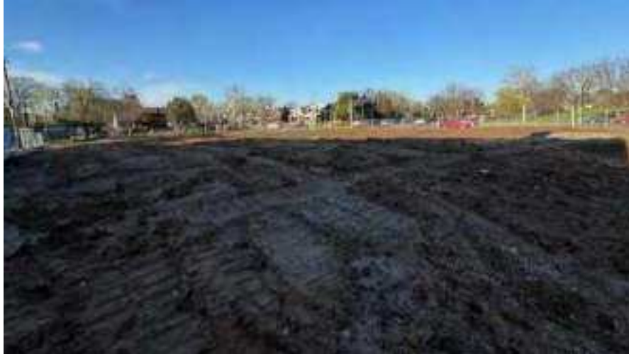
Site (After Demolition)
