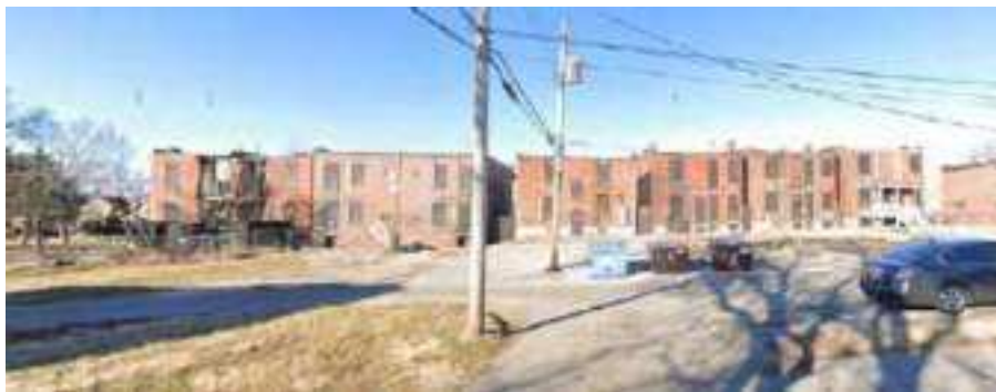
Back of Site (Before Demolition)
