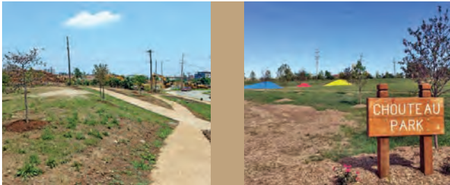
PHOTOGRAPHS OF CHOUTEAU PARK UNDER CONSTRUCTION
