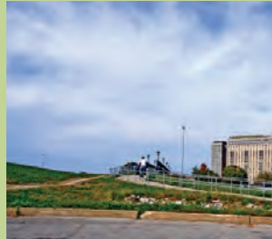
EXISTING PEDESTRIAN BRIDGE
