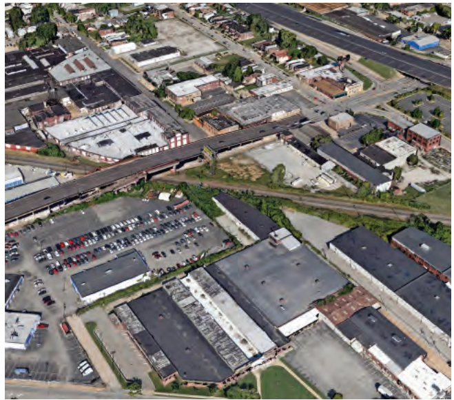
AERIAL IMAGERY OF KINGSHIGHWAY VIADUCT
