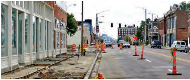
PHOTOGRAPH OF MANCHESTER STREETScape UNDER CONSTRUCTION
