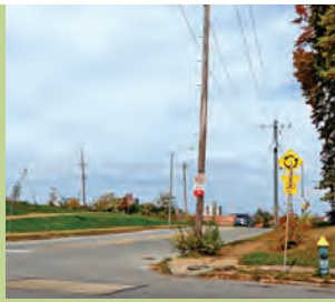
TOWER GROVE INTERCHANGE
