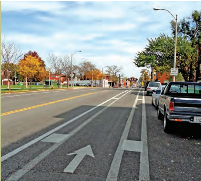
EXISTING BIKE LANE
